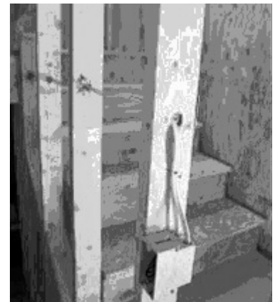
Nonmetallic sheathing helps protect wires from damage.
