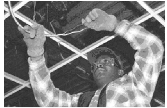
Electrical work can be deadly if not done safely.
