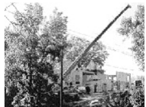
Operating a crane near overhead wires is very hazardous.
